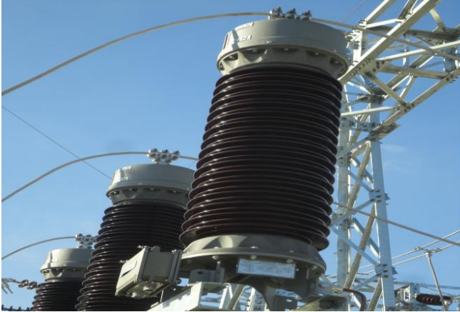
Figure1. Voltage Transformer used for 66kV in 230/66/11kV Substation.
